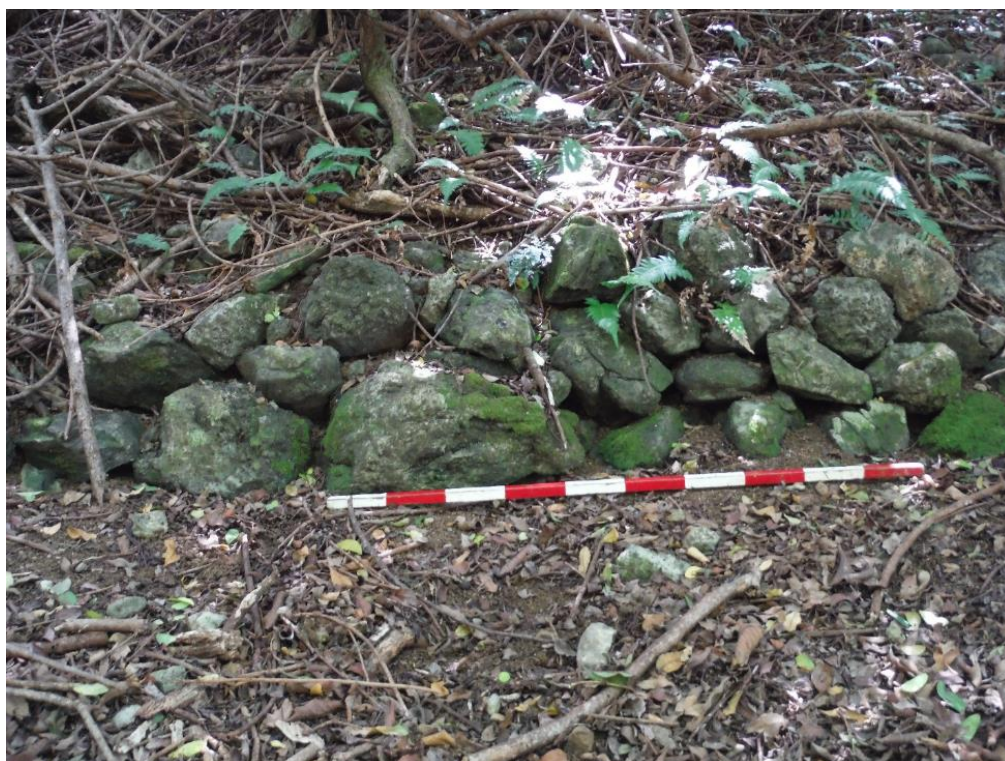
Figure 36. West retaining wall of feature WAI-4-W-Y, view to W.
