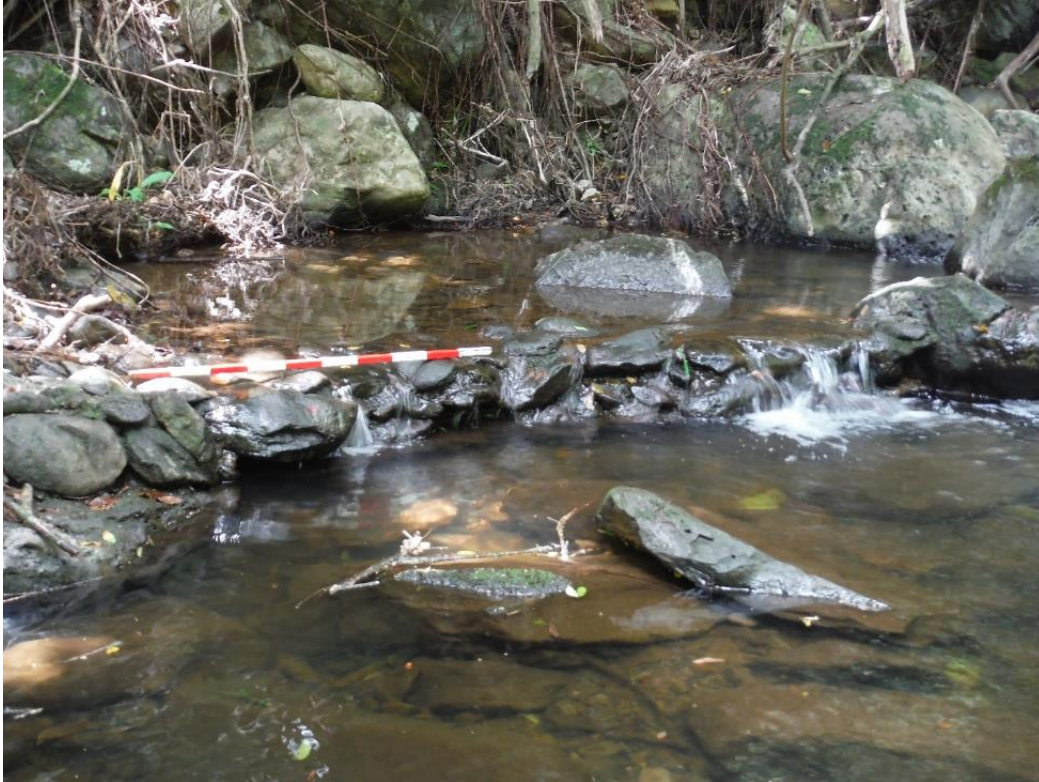
Figure 26. Concrete and stone Po'owai located South of WAI-2-S, view to SE.
