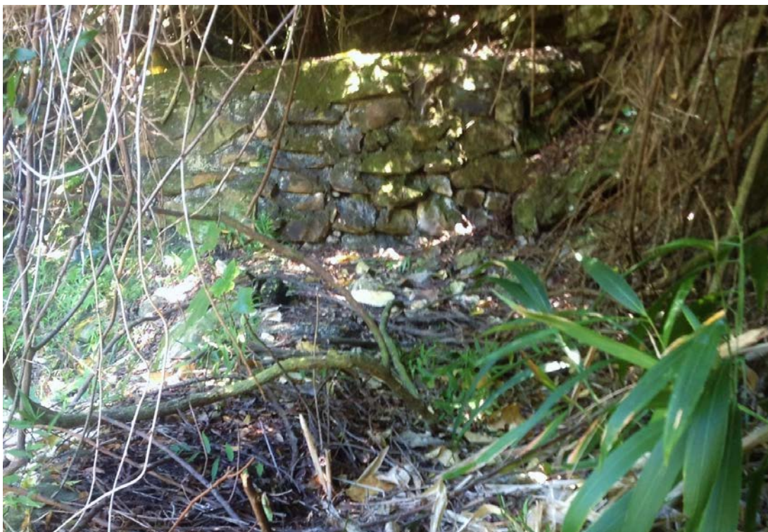
Figure 19. Photograph of barrier wall at east entrance to Wai'āpuka Tunnel.
