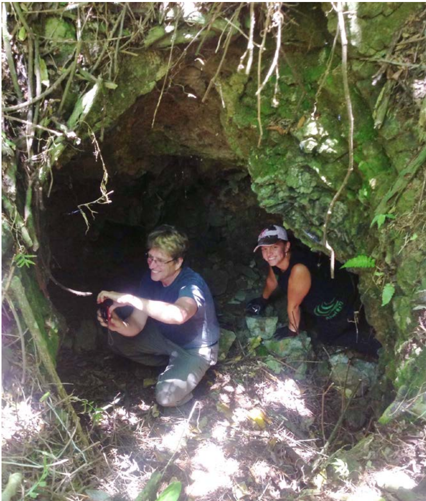
Figure 17. Photograph of a collapsed shaft associated with Wai'āpuka Tunnel, showing approximate diameter and depth.
